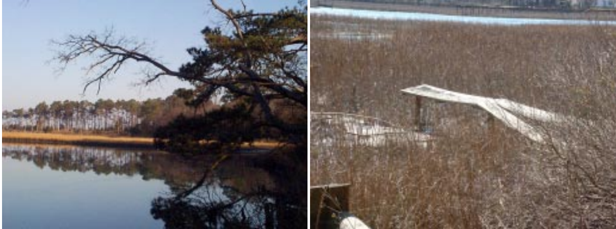
Sections of the footbridge that spanned Hoffler Creek remain in the marsh.
